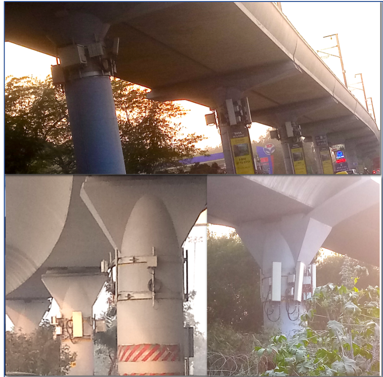
Figure 8: Antennas mounted on Metro Pillars
