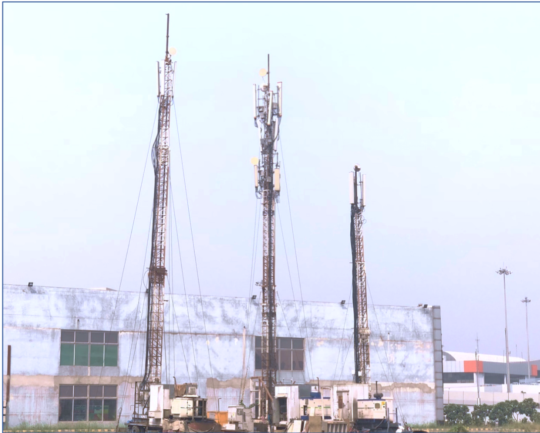
Figure 5: Cell on Wheels (CoWs) in front of T3 Terminal
