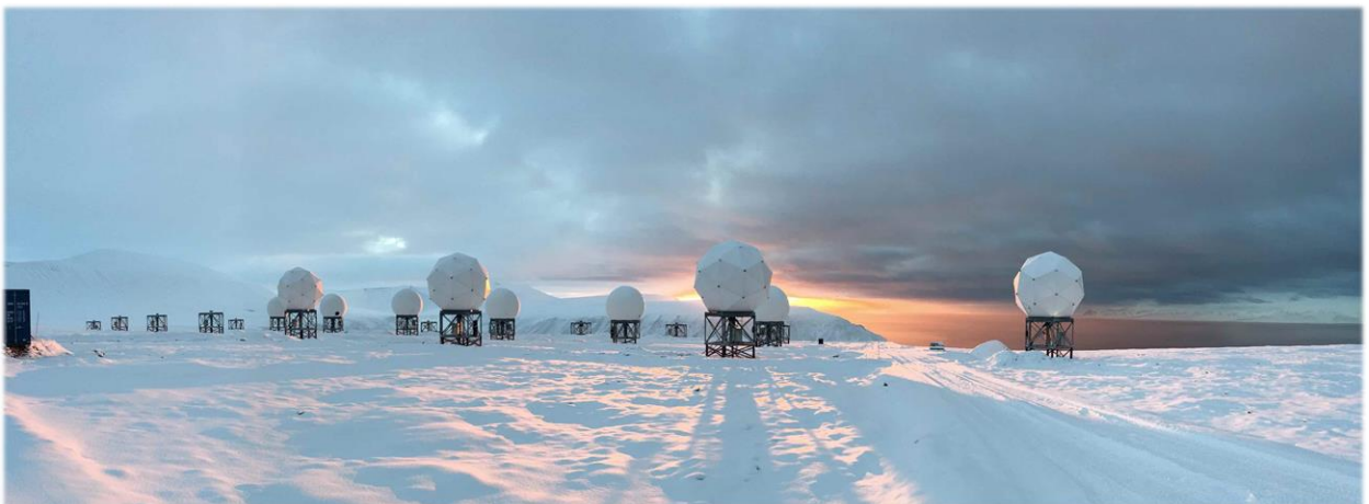
Figure: OneWeb Gateway Earth Station in Svalbard, Norway
